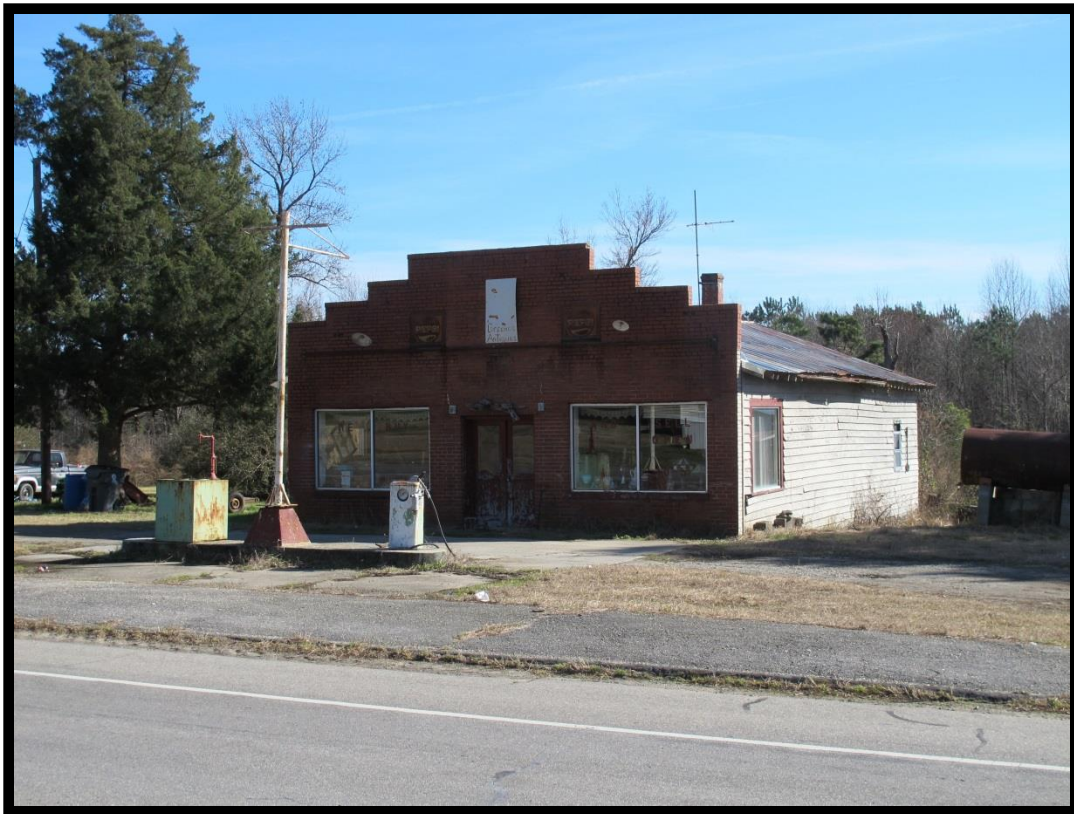
Figure 19: Sugg's Store, ca. 1940 (ED0888). Edgecombe County, South of the Intersection of Suggs Road with NC 258.
